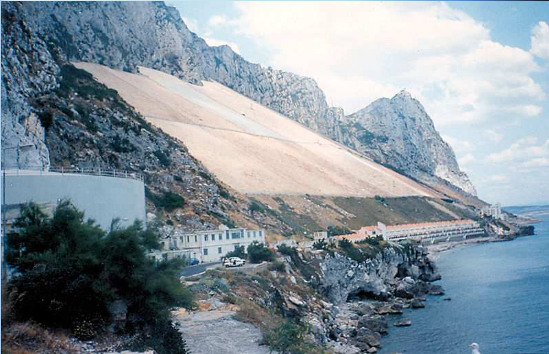
A water harvesting system collects rainwater from the Rock of Gibraltar into pipes which lead to tanks excavated inside the rock.
